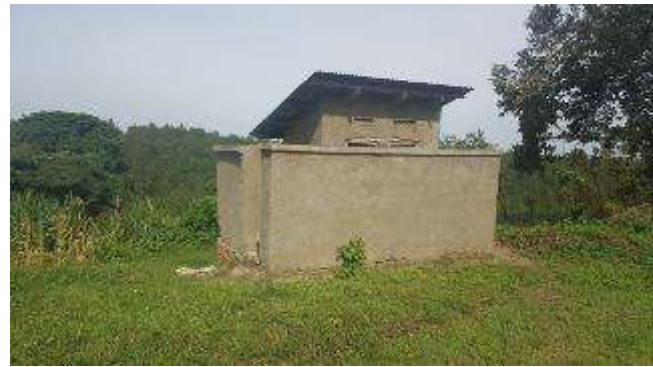
Latrine in Kihhi Town Council
